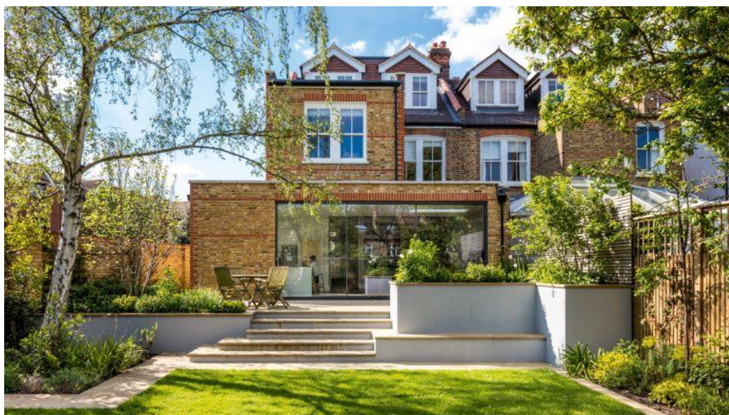
Figure 5: Contemporary/contrasting extension on a traditional style house built using matching brick with quoins, heads and banding detail to match the existing dwelling (Image credit: Grant Architecture and Interiors)
